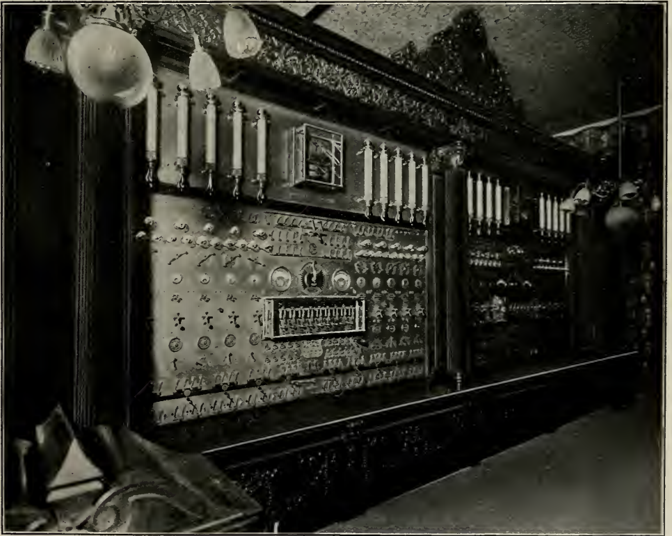
FIRE-ALARM SWITCHBOARD
